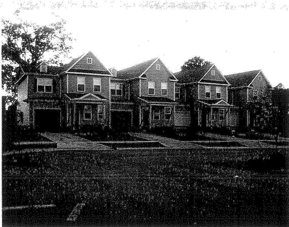
Bandolier Circle, 1357, All Support Beams Installed, 09/12/08
