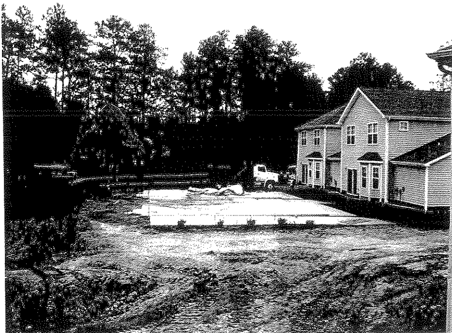
Virginia Place, HH-VP-34-36, Initial Demo Pad, Picture 1,
