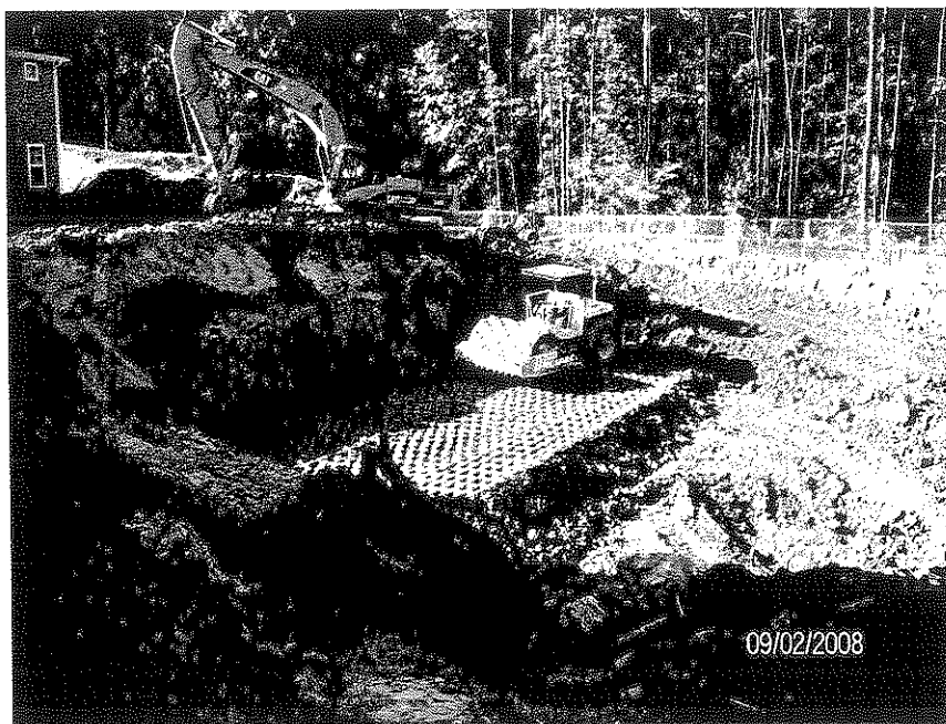
Virginia Place, HH-VP-34-36, Compacted Backfill, Picture 09
